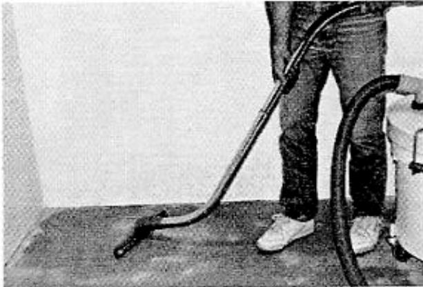
Vacuuming entire floor.
