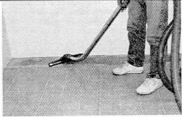
Vacuuming exposed floor after removing three strips of flooring.
